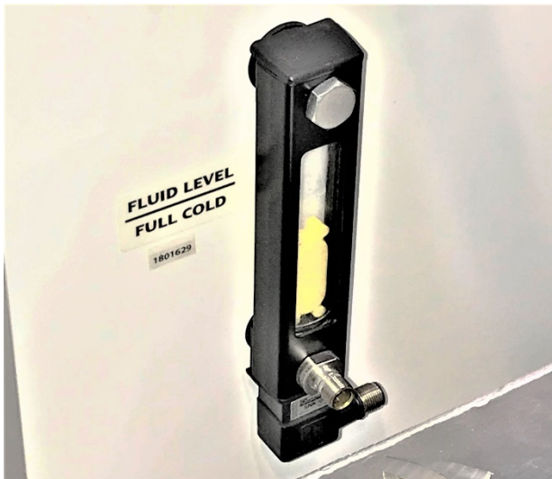
Hydraulic Reservoir Sight Gauge
