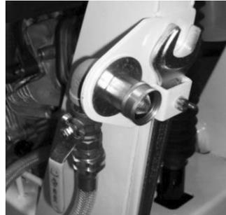
**Figure 17: Water Supply Fitting**
