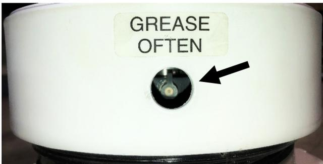
Upper Blade Shaft Bearing Grease Fitting Access
