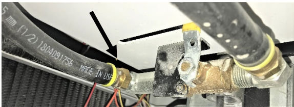
Water Valve Outlet Hose Connection
