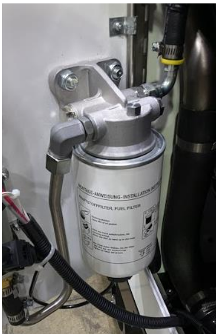
Fuel/Water Separator Filter
