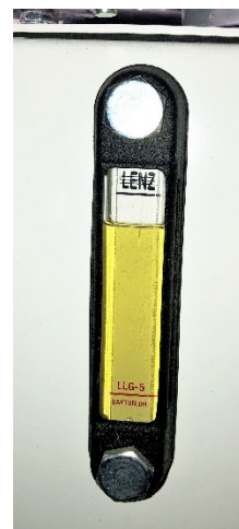
Liquid Level Sight Gage
